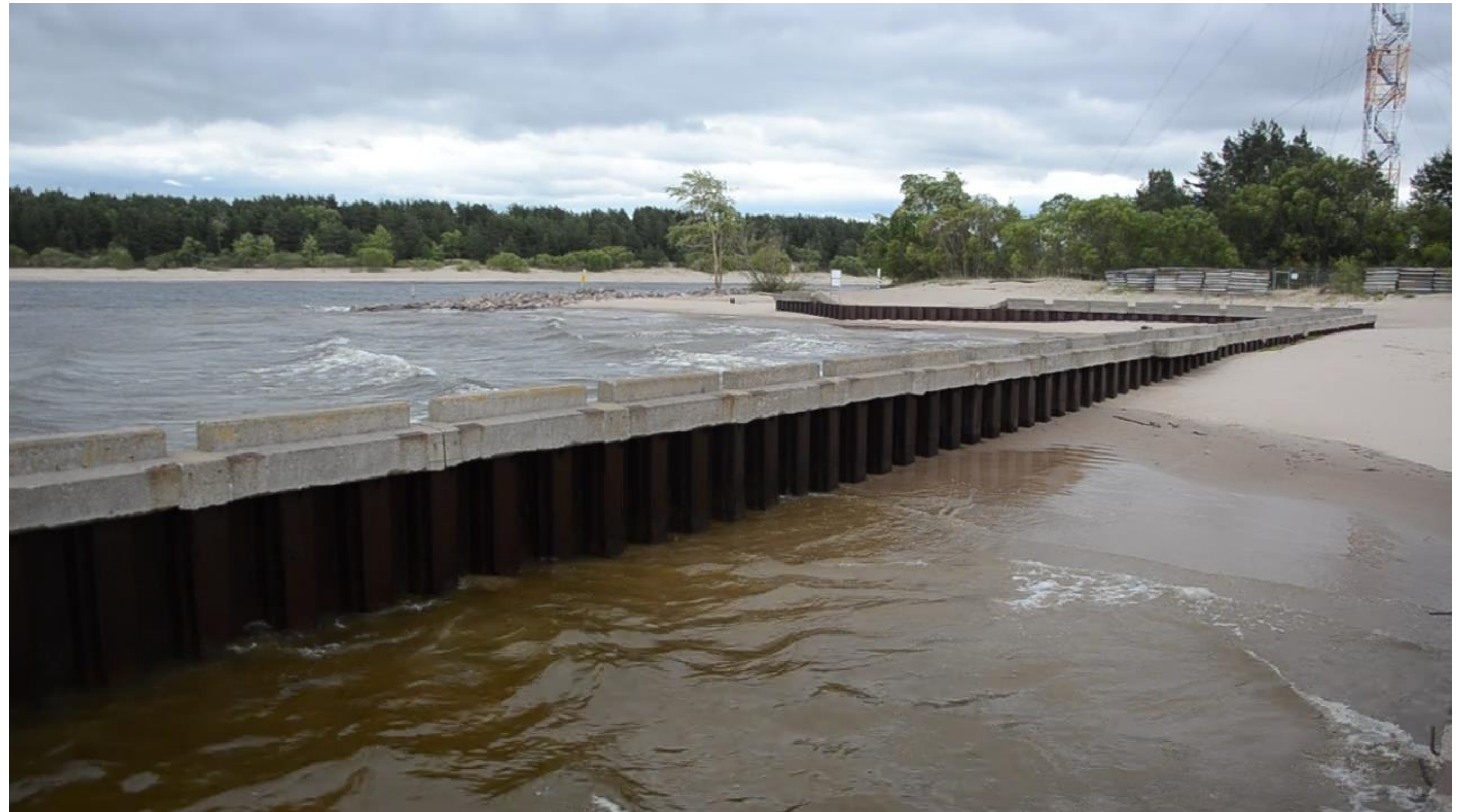
Current breakwater at Narva to be improved (video provided by Rain Mannikus)
